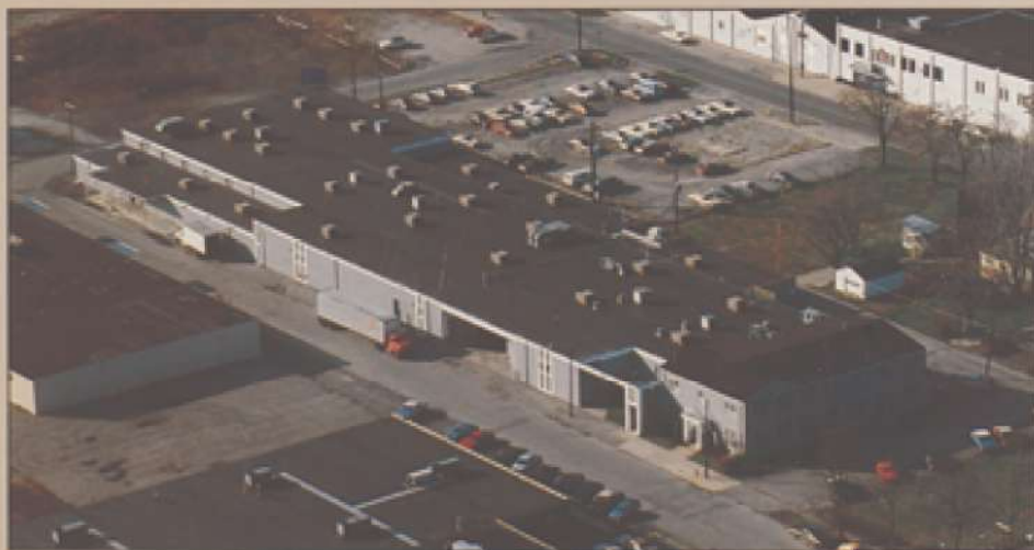
(Top) Plants 1 & 2—100,000 sq. ft. Plant 1 houses transformer/battery charger production. Plant 2 houses AC ballasts, DC ballasts and power supply production.
